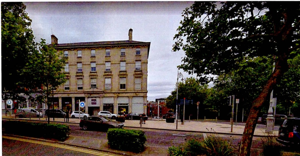
Figure 2.0 Street-view image of the subject site. We note that the car parking bay is fully occupied in this image.
